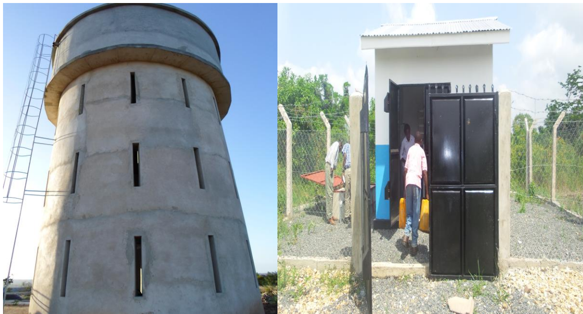
80 m 3 and 9m overhead tank and pump house constructed at Mpiji Magohe water scheme.
